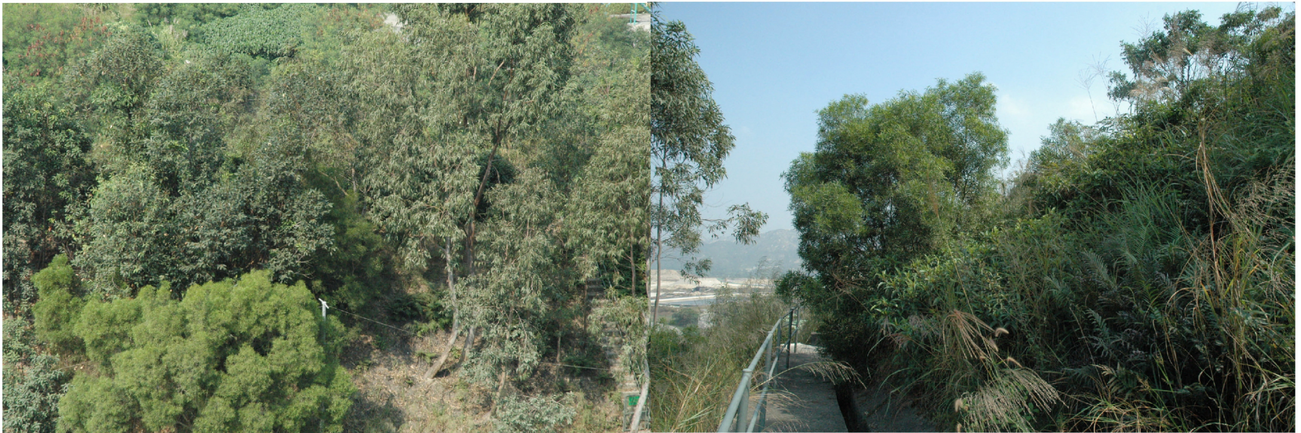
LR6 - SLOPE/REINSTATED PLANTATION
